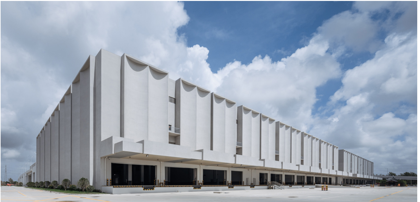
Lingang Warehouse | Shanghai, China
