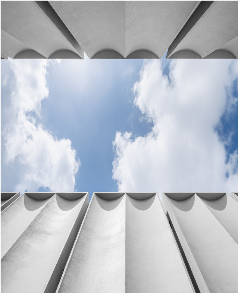
Lingang Warehouse | Shanghai, China
