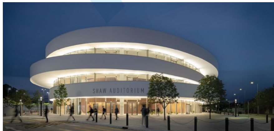
Shaw Auditorium | Hong Kong, China © Copyright Kris Provoost, courtesy of Henning Larsen Architects
