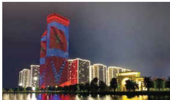
TECHNO PARK TOWER VINGROUP, HA NOI - 2021 FIRESHIELD
