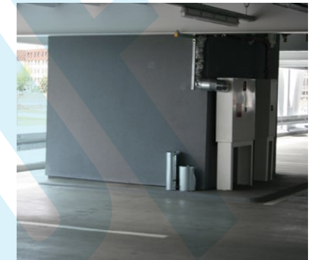
Car Park Utility Rooms | Stuttgart, Germany
