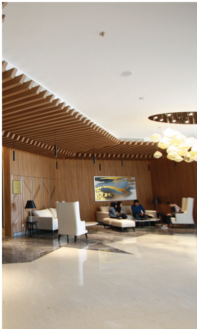
The Kensington Apartment Flat Ceiling
