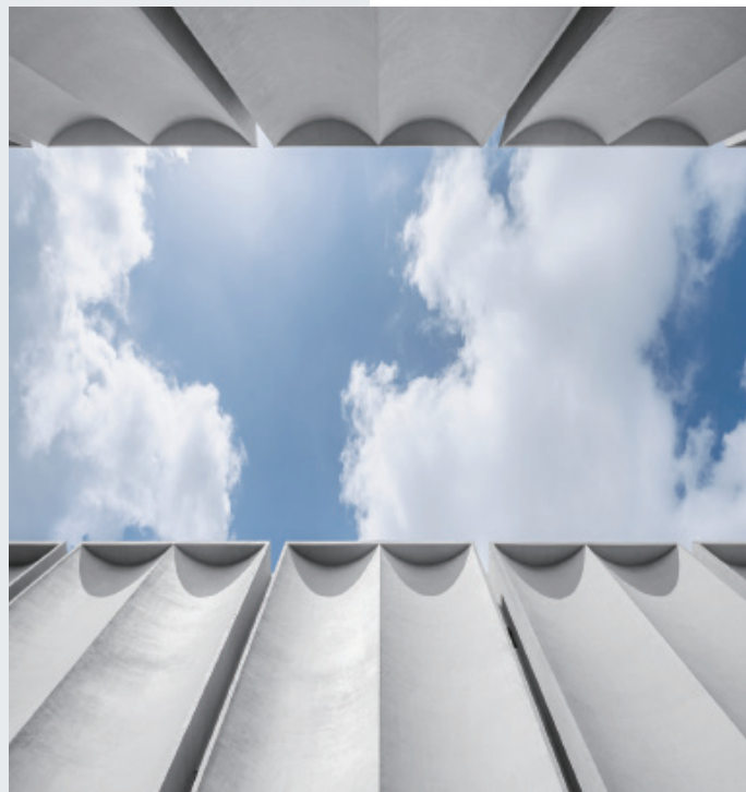
Lingang Warehouse / Shanghai, China
