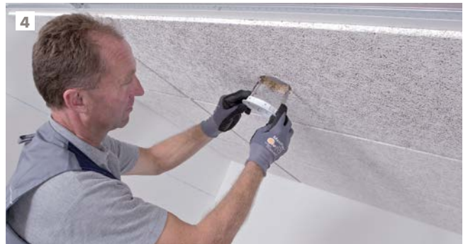
4 Insertion of the spotlight housing.
