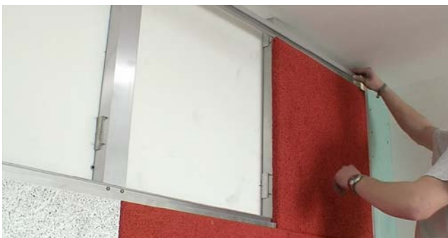
Installation of the upper edge profile. Space required from the ceiling approx. 40 mm. The first tile is moved approx. 10 cm towards the middle, the screws are fixed and then the tile is finally aligned in the grid.
