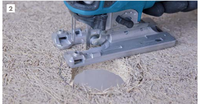
2 Cutting out an aperture with a jigsaw, tile face side down.
