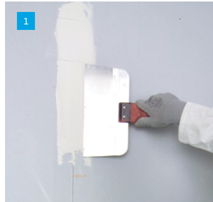
Applying Knauf Joint Filler Premium to either side of the corner.
