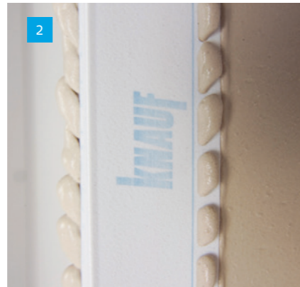
Ensure all holes are completely filled.
