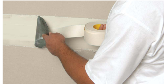
2. First coat – Bed tape
