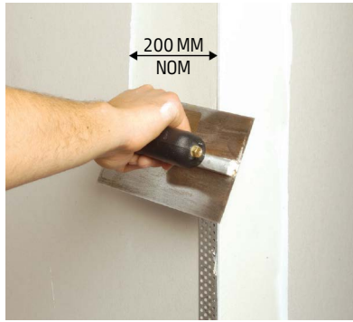
2. Apply first coat to both corner faces
