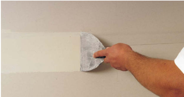
1. First coat – Bedding compound
