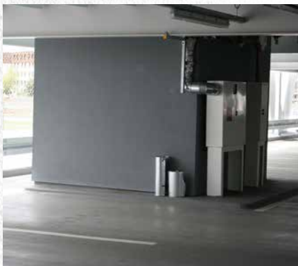
Car Park Utility Rooms | Stuttgart, Germany
