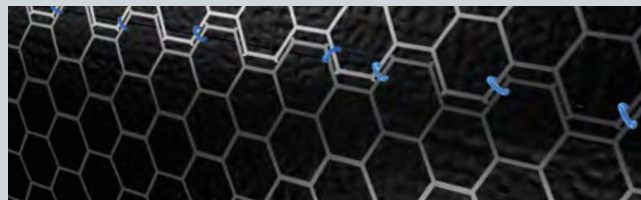
Picture 2: Binding wire loops
