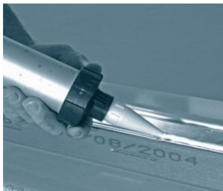
Apply Knauf Acoustical Sealant or Knauf Insulation strip. (optional)
