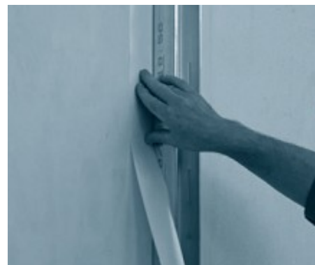
Alternatively, apply the Knauf Trenn-Fix on solid components or on drywalls after fixing the perimeter frame.
