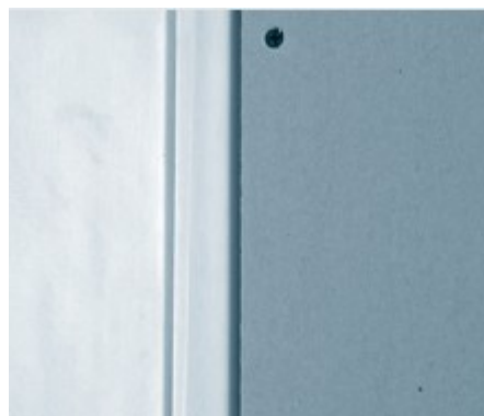
Leave 5mm jointing gap to install Knauf Gypsum Boards.
