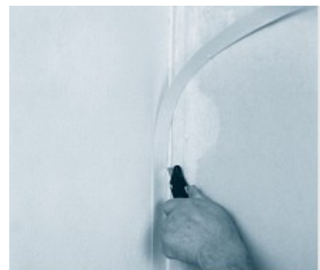
Trim the excess material once the joint filler dries off
