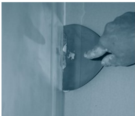
Fill the joints
