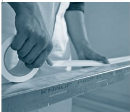
Apply the Knauf Trenn-Fix on the CW+, CW, UW or UD Profile.
