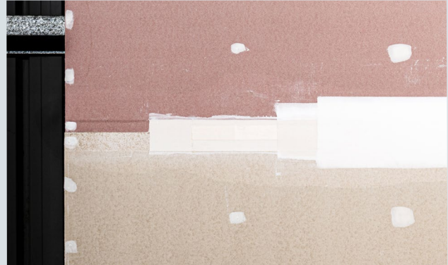
Figure 12: FIBEROCK Aqua-Tough and Plasterboard Setting Joints
