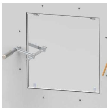
EN - Adjust the frame (check angularity), fasten it and mark the drill holes , Drill distance  $\leq 200$  mm.
