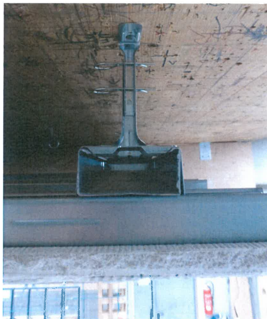
Figure 3: Detail: Nonious hanger Ceiling system "D282.de with AQUAPANEL Cement Board Indoor (Lighter.Easier.Faster.)"
