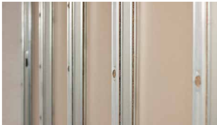
Attach any required Knauf MaxSpace traverses at the appropriate locations between the uprights with four quick-release parkers (length max. 10 mm).
