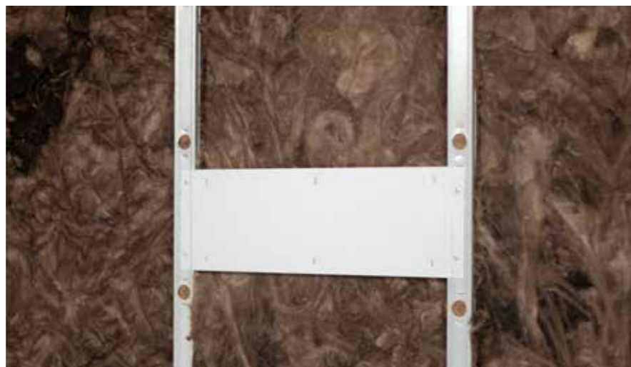
Attach any required Knauf MaxSpace traverses at the appropriate locations between the uprights with four quick-release parkers (length max. 10 mm).
