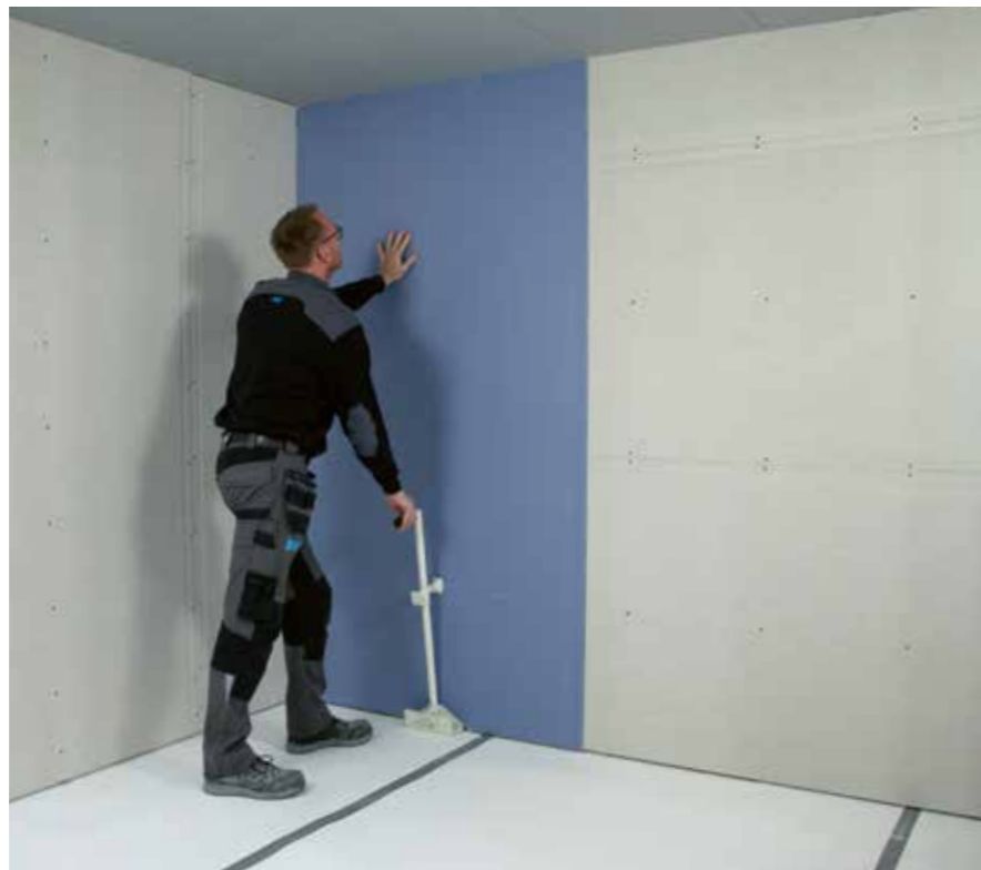
Application of Knauf Diamond Boards as second cladding.
