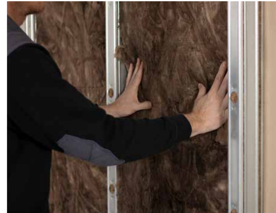
Application of Knauf Acoustifit between the uprights.
