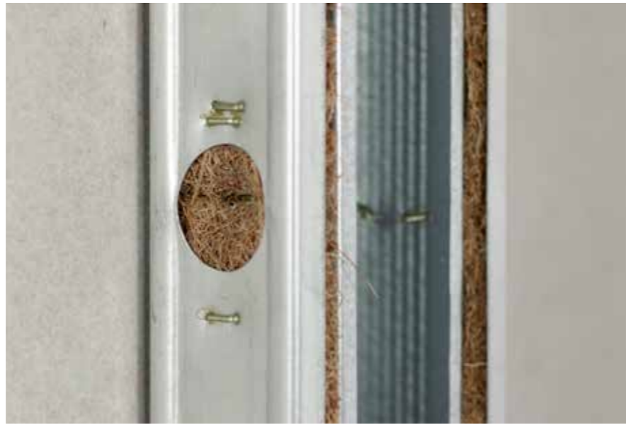
The wall will be clad on both sides with 12.5 mm Knauf A-board and 12.5 mm Knauf Diamond Board. The cavity space is provided with 60 mm of glass wool Knauf Acoustifit. The total wall thickness is 125 mm.
