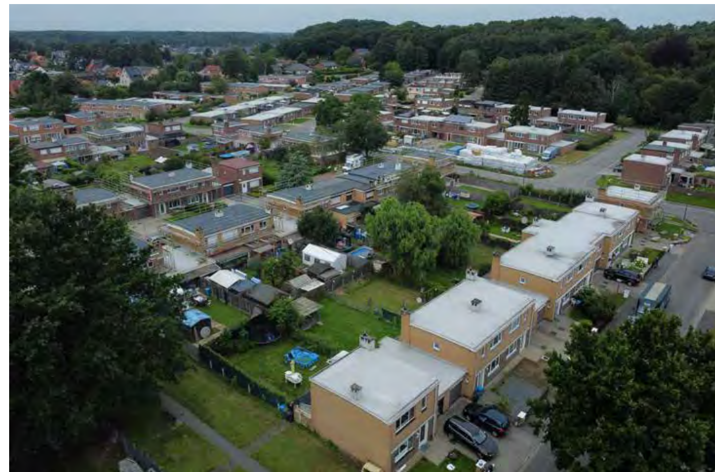
Work begins in Aarschot on the second biggest Knauf Energy Solutions initiative in Belgium
