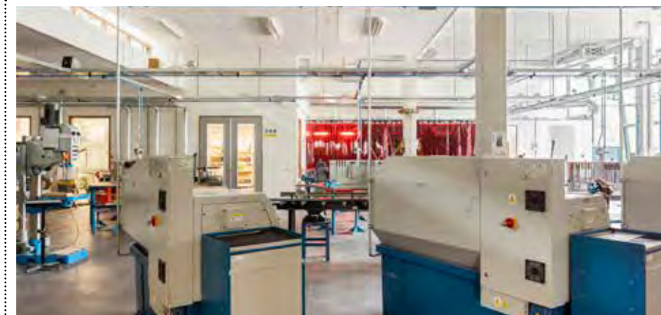
Heraklith A2 Wood Wool was installed in Da Vinci College in the Netherlands to minimise noise from adjoining classrooms
