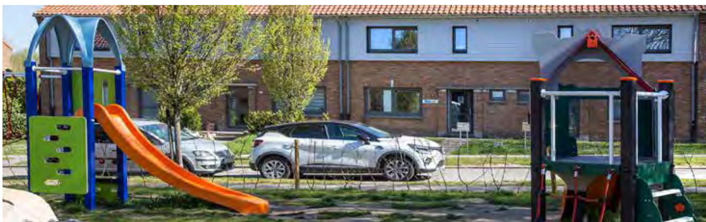
KES provided a range of energy renovation options to meet the needs of the housing association
