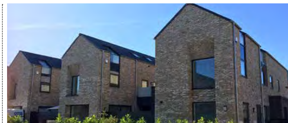
Knauf Insulation's Acoustic Roll and OmniFit Roll were installed in The Gables housing project Liverpool, UK to achieve great levels of thermal and acoustic comfort
