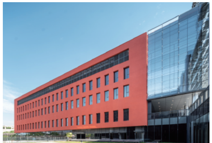
Hunan Broadcasting System Program Production Center China
