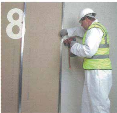
8 Fixing Knauf Plasterboard to the completed framework.
