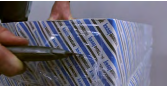
Cut the plastic wrapping by running a knife along the sides of the package. Do not cut the plastic on top of the package.
