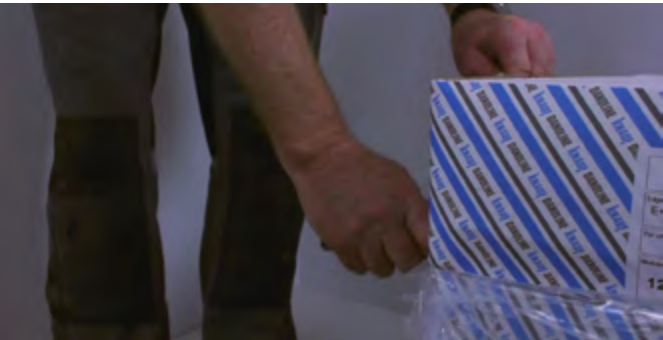
Remove the cardboard liner around the ceiling tiles.
