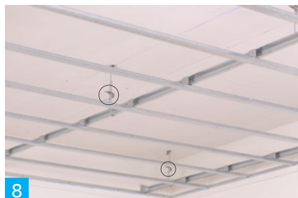
5 Build the hanging set by bending the end of the Hanger Wire then assemble with KC50 Adjustable Spring and KC50 Hook Wire. Then install it to the Bolt Angle.
