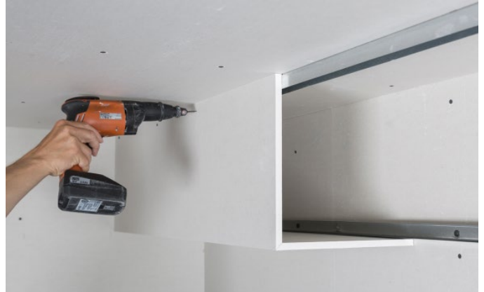
Image 3: Screw fasten the Klebe-Fix
