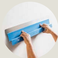
Skimming - Enduisage complet (F2b/F3)
