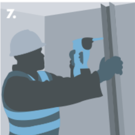
7. Fixing Knauf Deep Flange 'U' Channel to studs at door opening.
