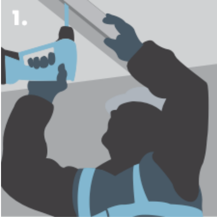
1. After fixing the head track, the floor track should be positioned by using a vertical stud a laser/ spirit level.
