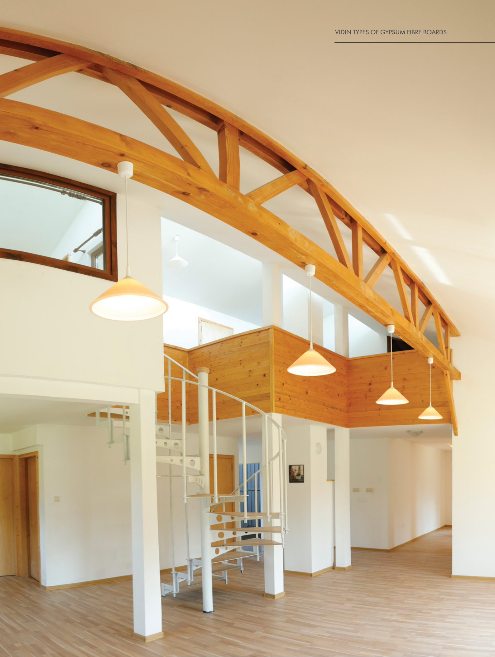
Single-family residential building with timber structure and Vidiwall boards
