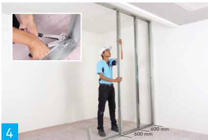
4 Install the C Stud in to the installed U Track by insert it in and adjust to make it be vertical to U Track, then fix them together with 13 mm truss head screw or using Metal Stud Crimper. Each stud should be 600 mm apart from each other and not less than 150 mm.
