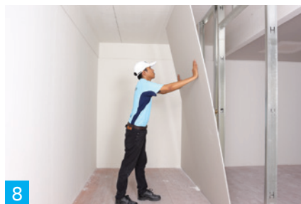
8 Install a gypsum board alternatively to the opposite side of the metal profile. Start from install the 600 mm wide gypsum board following by 1200 mm.
