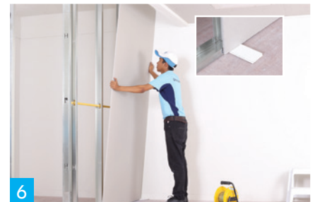
6 Before installing the gypsum board, lift the gypsum board up for about 10 mm (using a left-over gypsum board as a bolster is recommended for more convenience).
