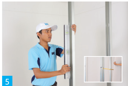
5 Install the rest of C Studs and have them all face to the same way. In case of the wiring is required, insert the wire through the H-shape hole on the stud first before install a gypsum board.
