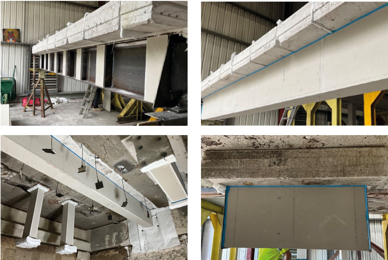
Figure 3: Photos of Knauf Fireboard being installed at a UKAS-accredited test centre
