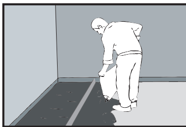
Level flattening - dry fill (if necessary) and gypsum plaster board
