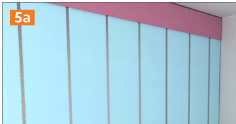
Step 5a: OPTION 1: Over-Partition Installation - Seal Perimeter (Outer linings at ceiling level)
