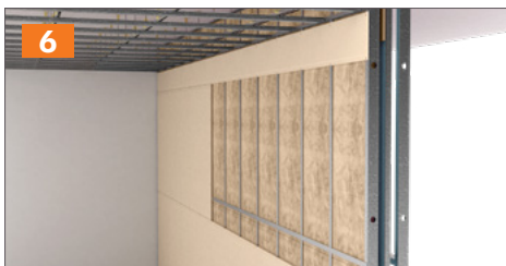
Step 6: Framing Installation
