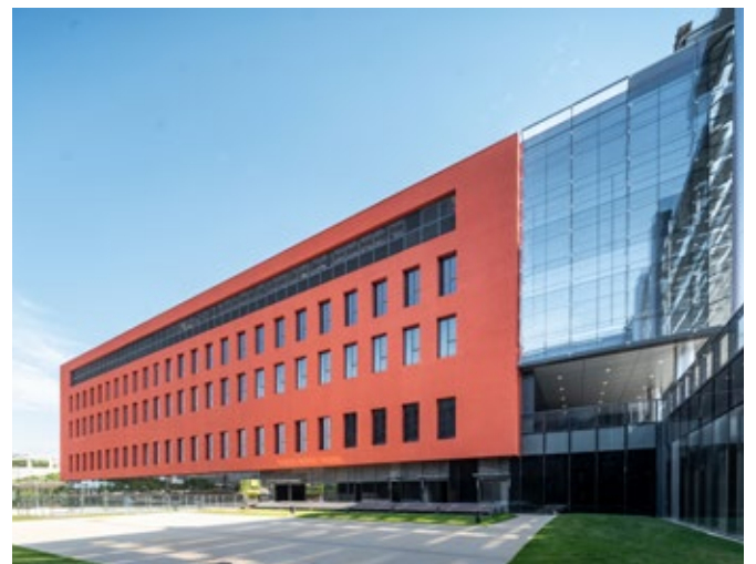
Hunan Broadcasting System Program Production Center | China
