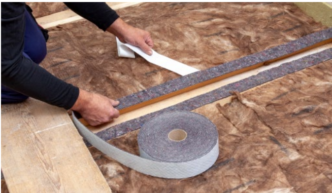
Bild 7: Fix GIFAfloor support insulation strip to the line-bearing.
