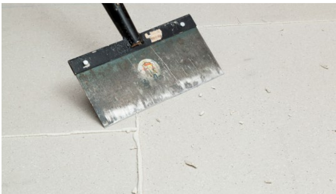
Bild 23: Remove any leaked adhesive the following day.
