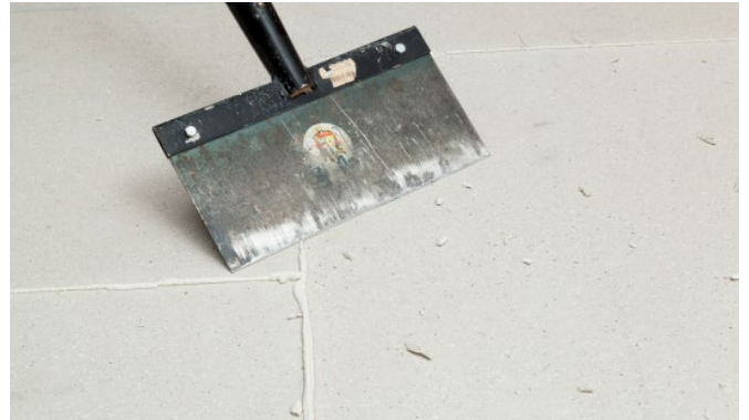
Bild 14: Remove any leaked adhesive the following day.
