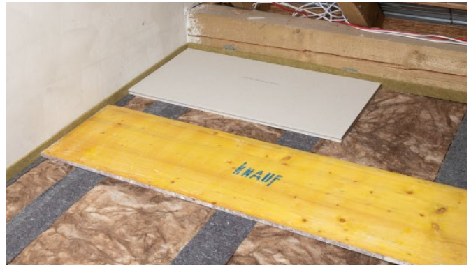
Bild 9: Install the cut-to-size GIFAfloor PRESTO floor element in the wall connection area.
