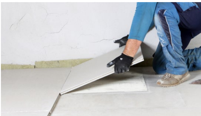
Bild 17: Laying GIFAfloor PRESTO elements in adhesive bed.
