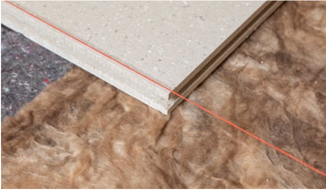
Bild 11: Cutting the wall connection element using a hand-held circular saw and GIFAtool Diamond saw blade.
