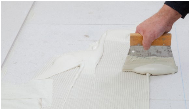
Bild 16: Spread GIFAbond duo EC 1 using a notched trowel.
