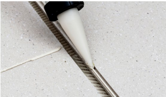
Bild 12: Bonding of tongue and groove connection.
