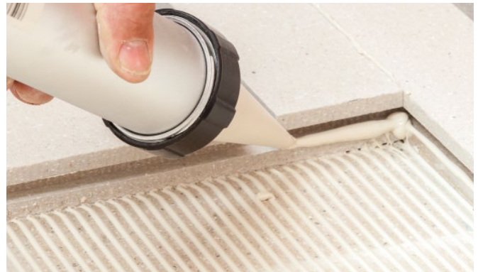
Bild 19: Application of adhesive to top of tongue.
