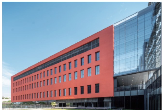
Hunan Broadcasting System Program Production Center China
