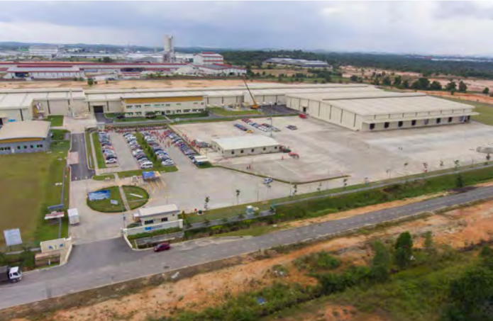
Glass Mineral Wool plant at Johor Bahru in Malaysia
