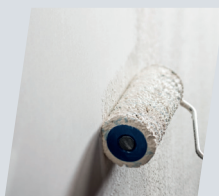
Skimming - Enduisage complet (F2b/F3)
