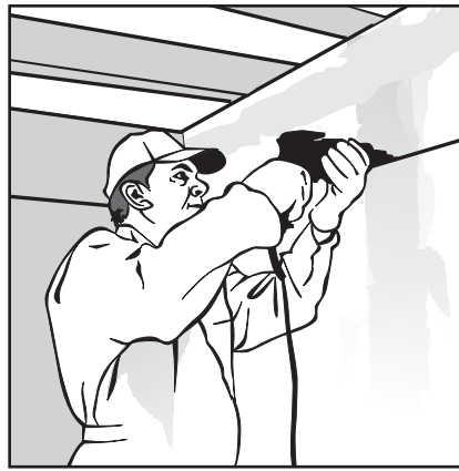
1. Fixing the perimeter L-channel
