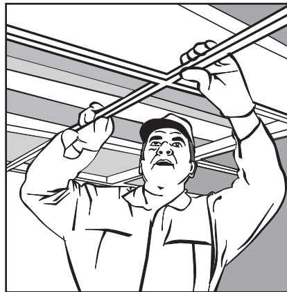
3. Installing the suspended grid
