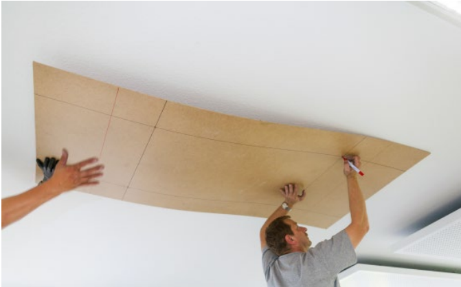
Image 4: Transfer of the suspension points
