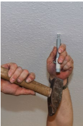
Image 6: Installation of the anchors/fasteners
