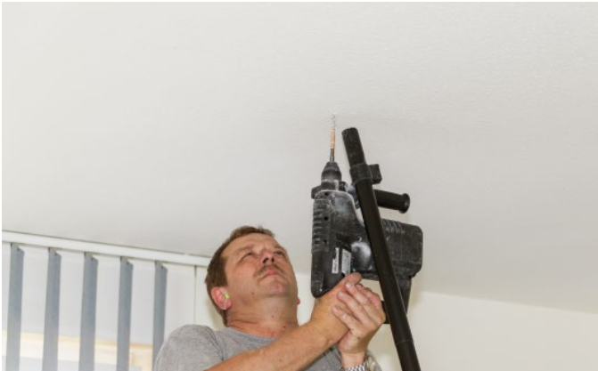
Image 5: Drill the holes for the suspension
