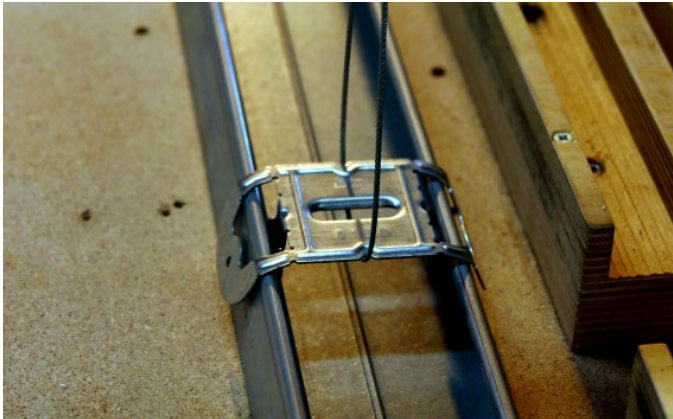
Image 10: Wire cord passed under the direct bracket
