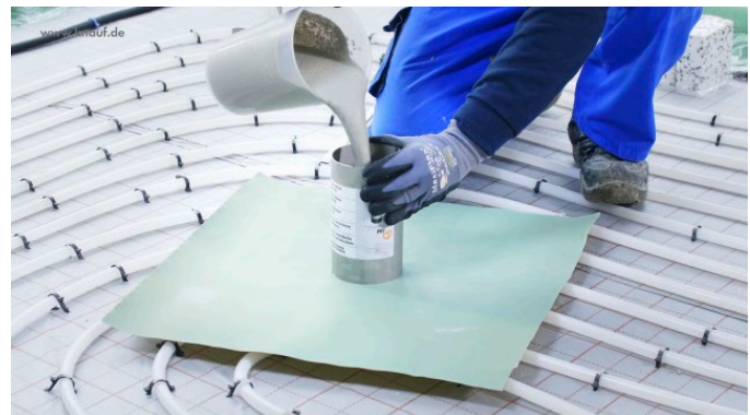
Image 2: Fill the consistence checking tin with mortar
