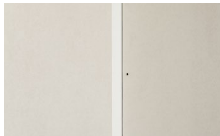
5. Install gypsum boards with 5 mm clearance
