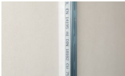
4. Push on the Trenn-Fix and smooth it
