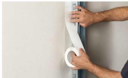
2. Attach Trenn-Fix beside the profile
