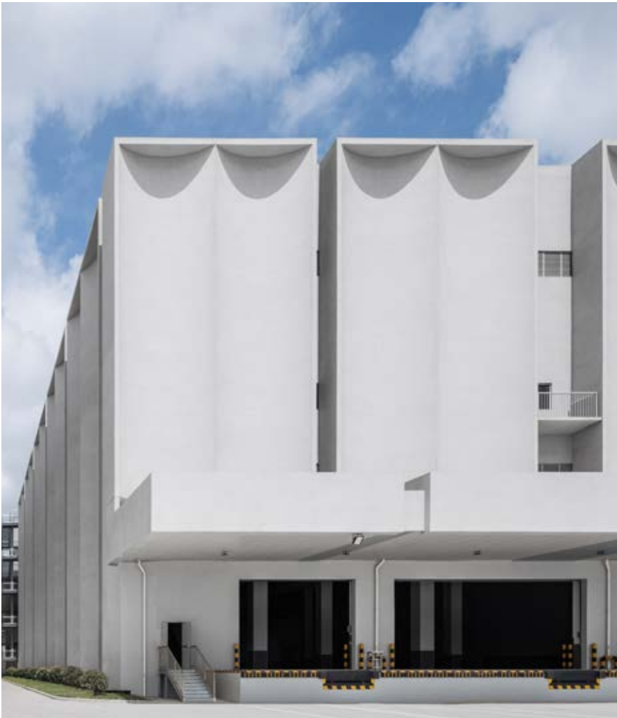
Lingang Warehouse | Shanghai, China
