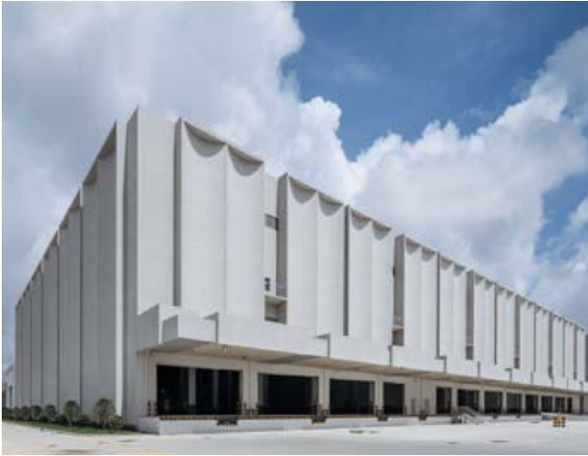
Lingang Warehouse | Shanghai, China
