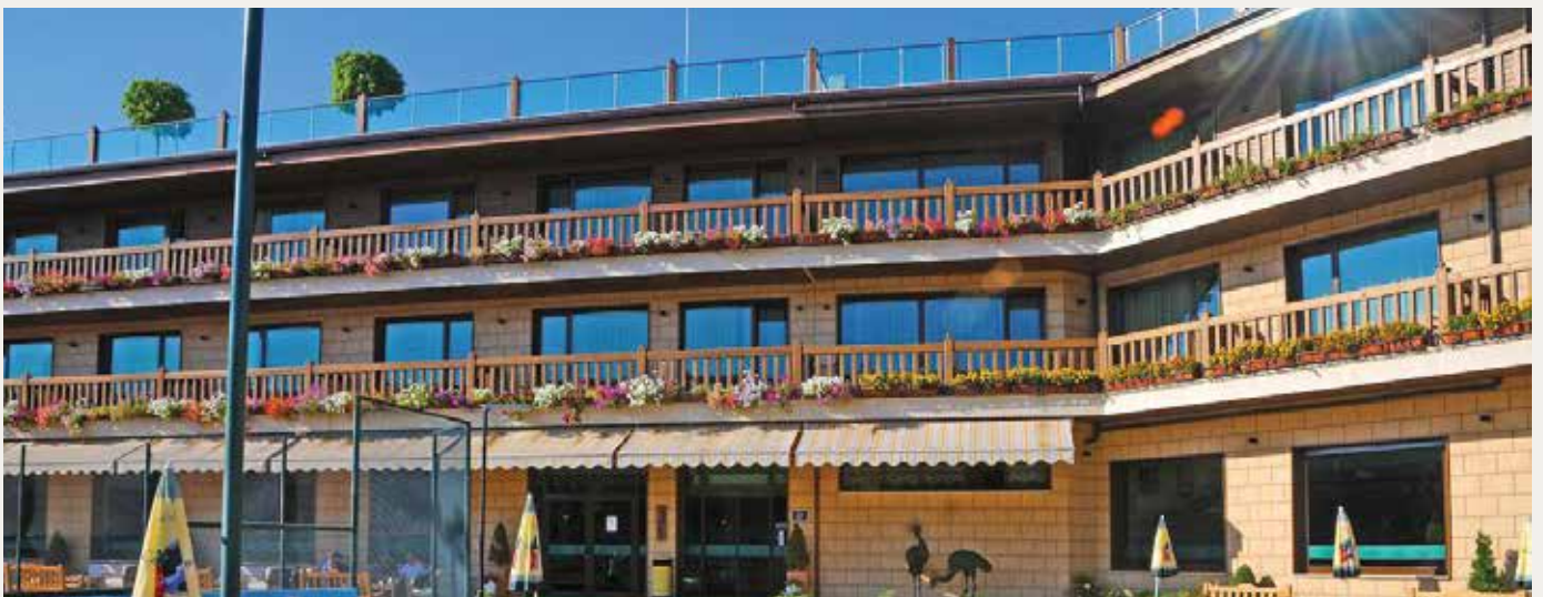
Hotel Izida, Dobritsch - Suchá podlaha F134 Vidifloor SOLO
