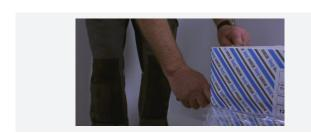
• Remove the cardboard liner around the ceiling tiles.
