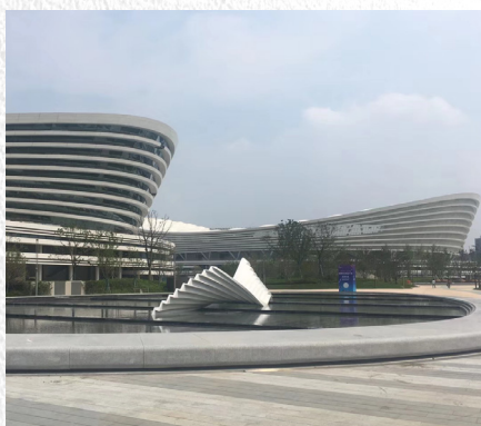
Suzhou Olympic Sports Centre | Suzhou, Chine
