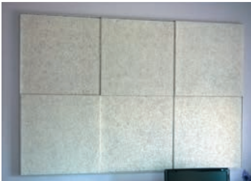
Position the panel in the frame pressing it against the support
