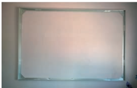
Position and attach the remaining profiles
