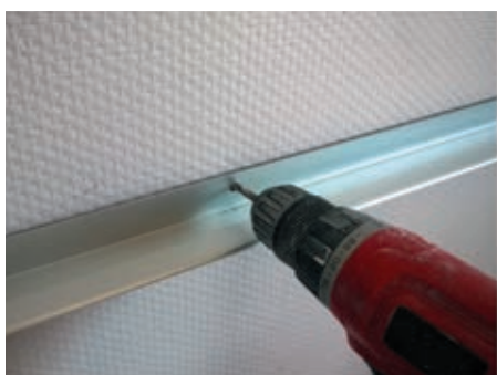
Position the 1,200 profile on the line and drill the 3 holes
