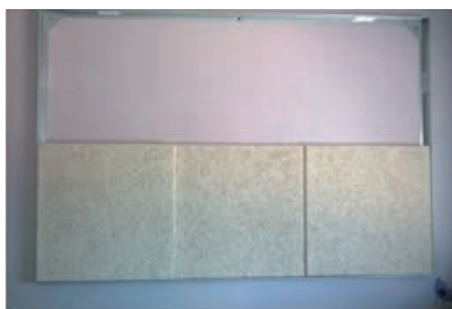
Position and attach the remaining panels
