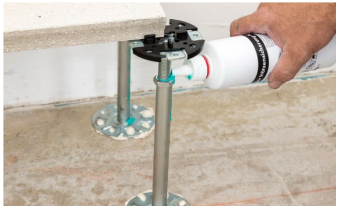
Bild 14: Installing the hollow floor element in the wall connection area
