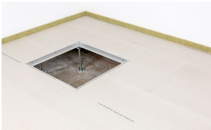
Bild 20: Installed access frame
