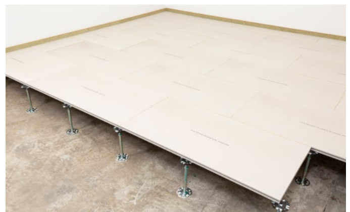
Bild 19: Installation of further hollow floor elements
