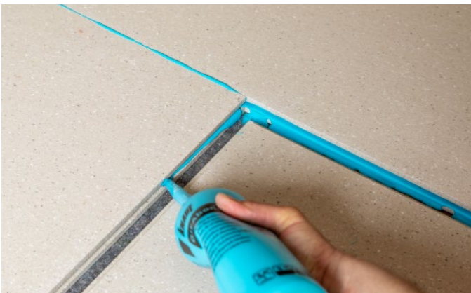
Bild 16: Application of adhesive.
