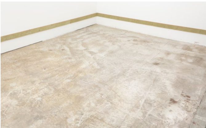
Bild 7: Fasten GIFAfloor edge insulation strip circumferential to wall
